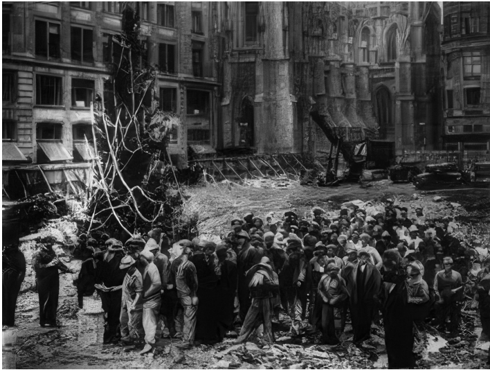
Dressed in overalls and jackets, wearing work boots and hats, Italian workers line up on Christmas Eve 1931 at the site of Rockefeller Plaza for that week's pay at the Midtown Manhattan construction site. Many of them chipped in to purchase the first Christmas tree at the site, which has become an annual tradition.
